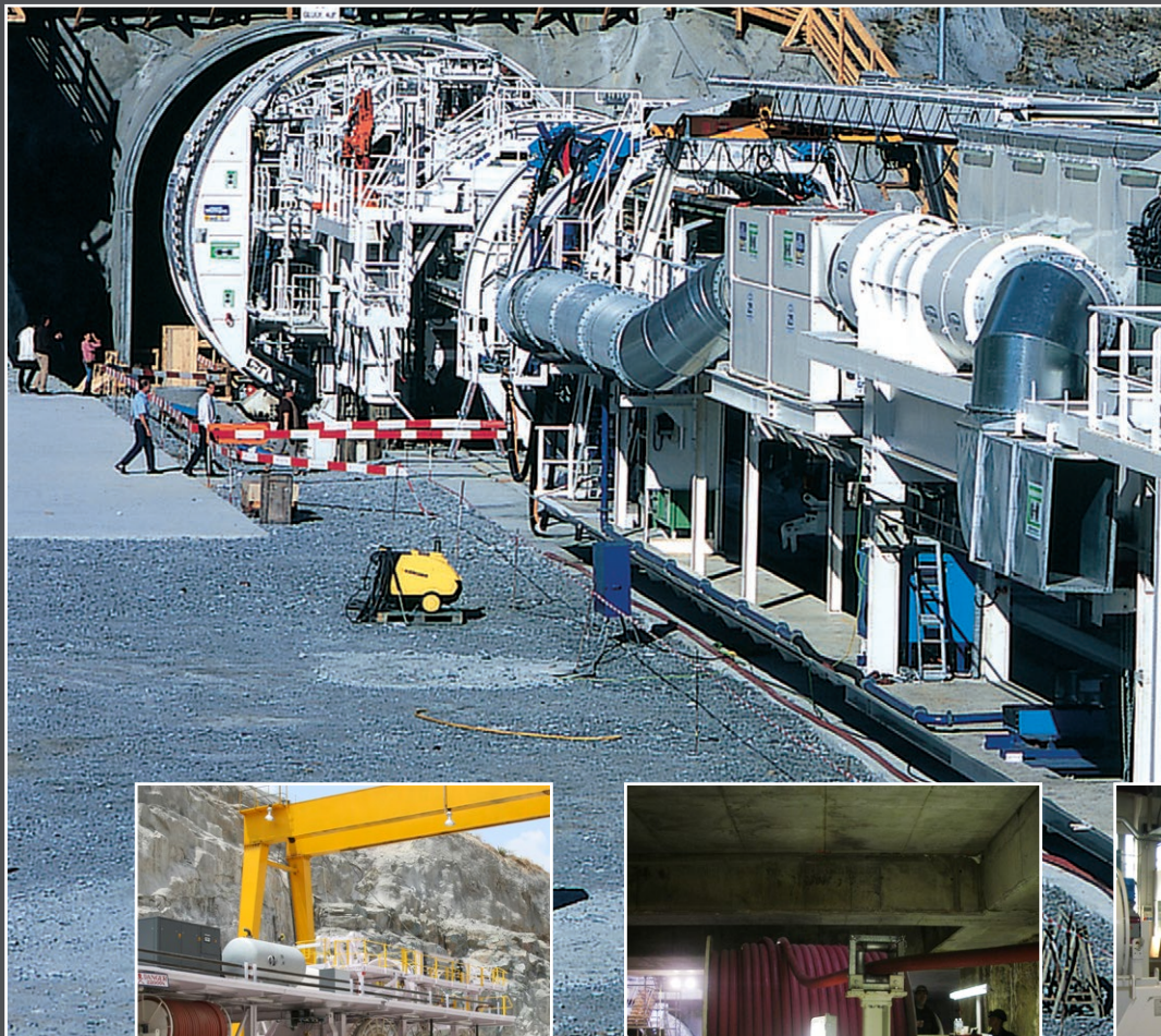
Orion cable reel with external slipping on Herrenknecht TBM
